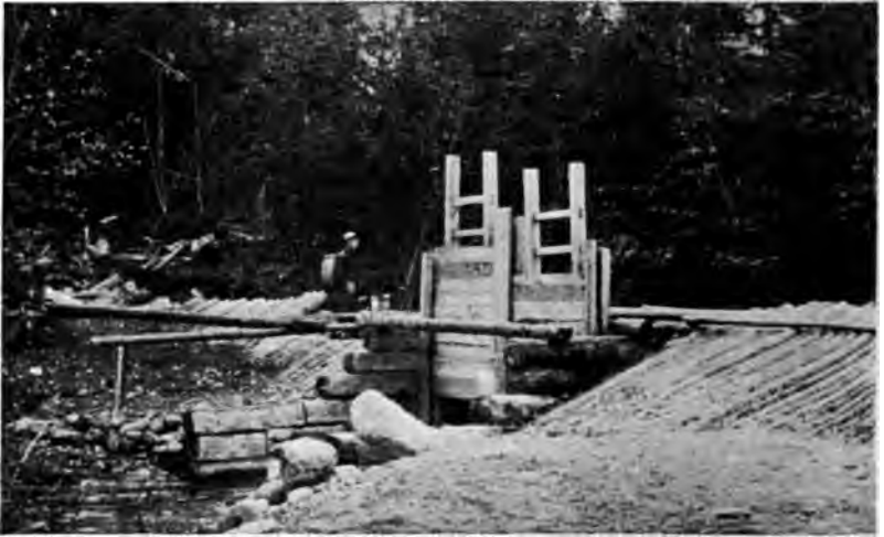
FIG. 100. — The Upstream Face of a Small Rafter Dam, showing a Common Form of Lift-Gate.
